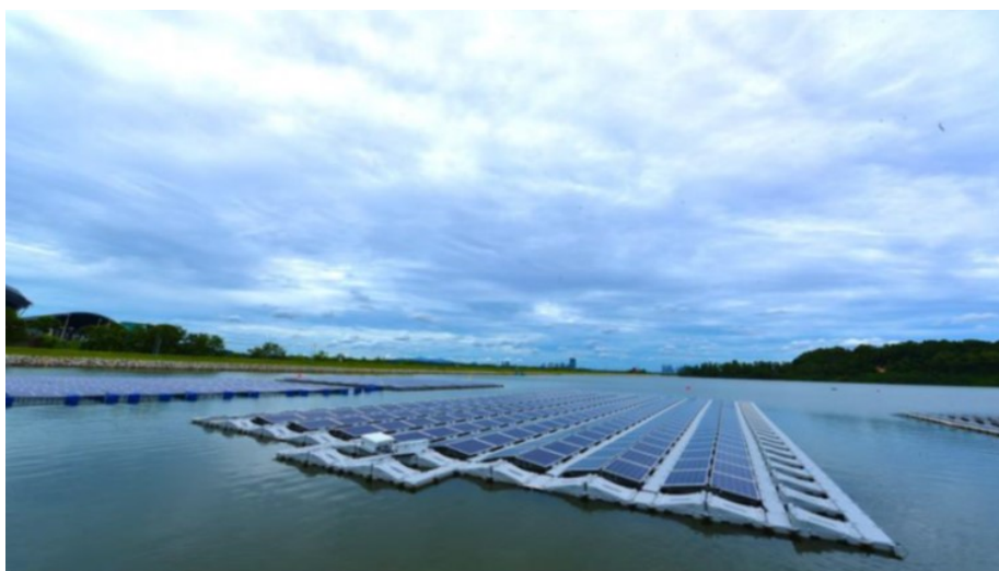
The one-hectare floating solar PV test bed on Tengeh Reservoir.
