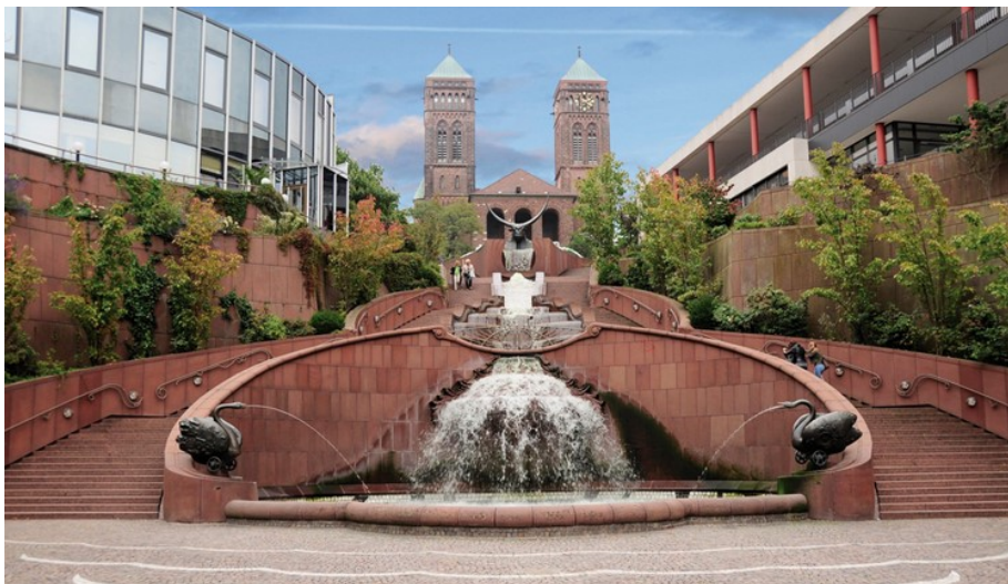
The city of Pirmasens in Germany provides district heating to hundreds of customers by sourcing heat from a combined-heat-and-power gas turbine, conventional heat boilers, and a waste incineration plant.
