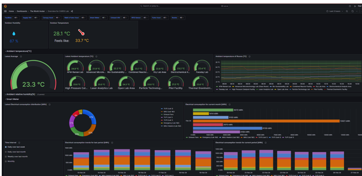
Figure 5.3: The CARES Laboratory Grafana dashboard for day-to-day monitoring of the laboratory conditions. It integrates data from a variety of sources, including an outdoor weather station, the laboratory's Building Management System, and an electricity meter to facilitate holistic monitoring of the laboratory operations.
